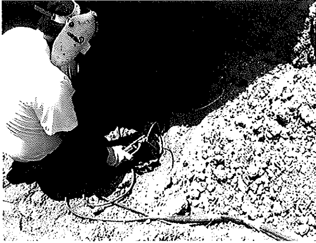
11 Top photo is a CP Tech tacking the wires and clips to the pipe after removal of the mortar diaper.. The bottom photo is a close-up of the leads from the pipe to the anodes.
