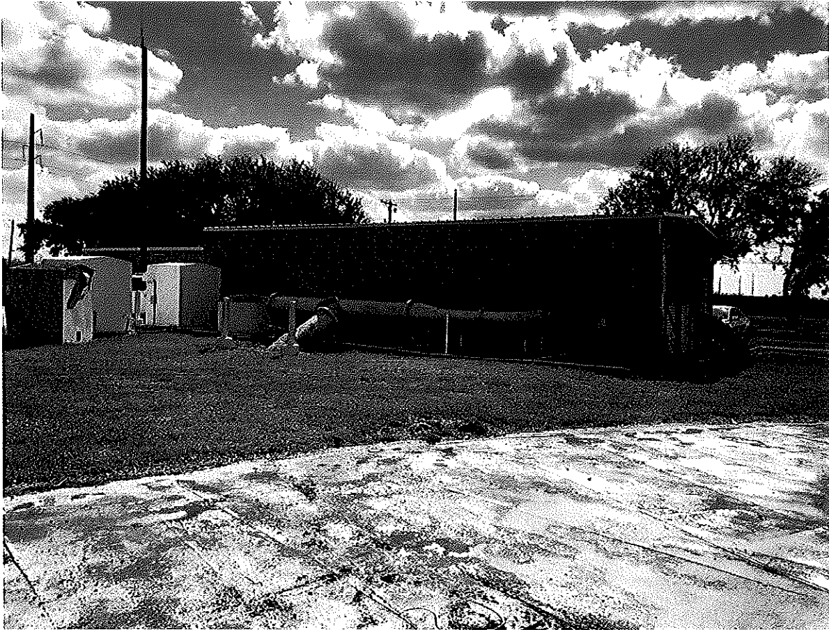
8 - Kingsville PS and Office Building in the background. The GST and PS equipment were conveyed to the City as part of the Water Supply Contract.
