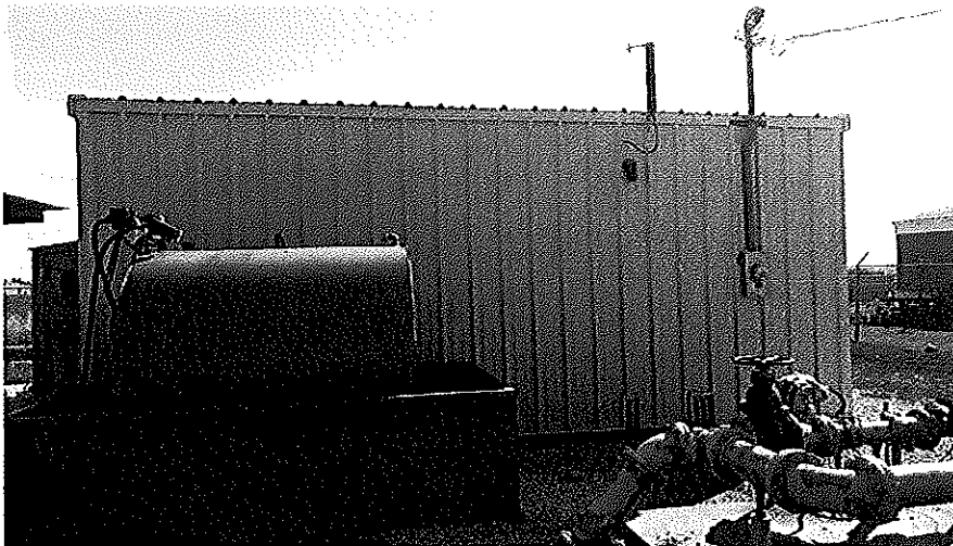
2 - Pump Station (PS) has been rehabilitated with a new exterior. All STWA pump stations have been rehabilitated with new exteriors.
